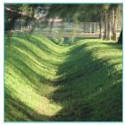
Edgewater's drainage is considered an open swale system. It is slow moving and designed to store and direct water to flow through it, while removing pollutants from entering ground water, ponds, lakes or the Indian River. It is not unusual for swales to hold water for several days after heavy rainfall. However, if water is standing in roads and sidewalks or water remains in swales longer than 72 hours after the last rain, please contact Environmental Services.
